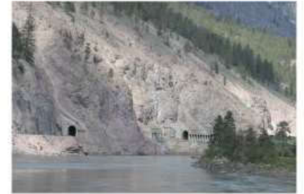
Rockfall and avalanche shelters over a railway line at the toe of a steep mountain slope.
