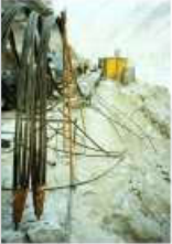
Drilling long holes for cables and installing a cable in a concrete buttress.
